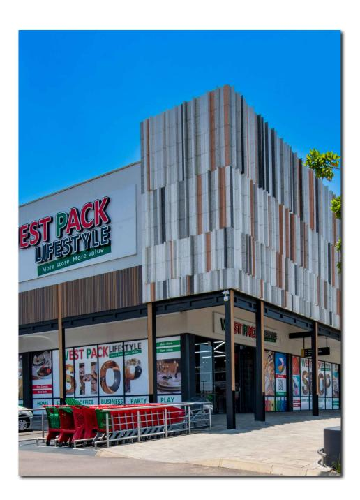
Lifespan architectural beams, with the UV-resistant Eva-tech finish, in the subtle Savanna colour, added an organic, warm, and welcoming ambience to the mall's entrance and walls, simultaneously providing much-needed shade from the sun. Their protective exterior coating echoes the natural shades of the environment and additionally provides a scratch, fade and insect resistant surface that withstands the climate whilst maintaining their appearance.
